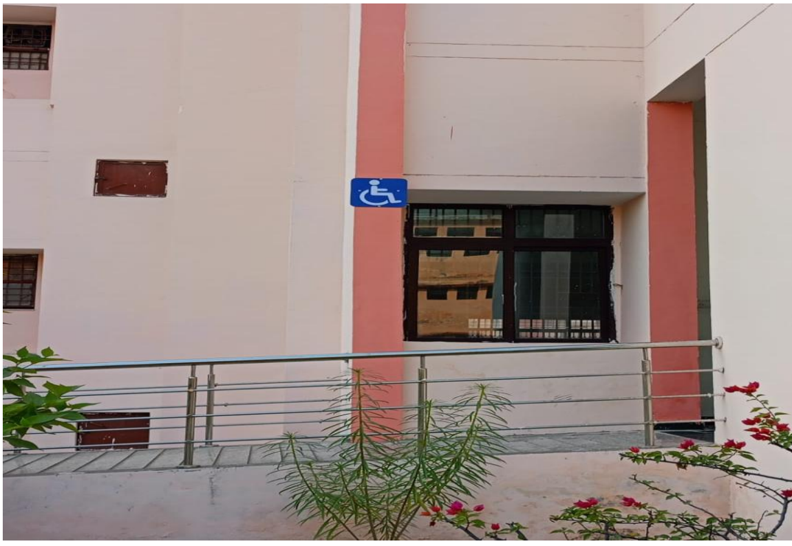
Figure 3.5.1(b): Ramp in the Faculty of Science
