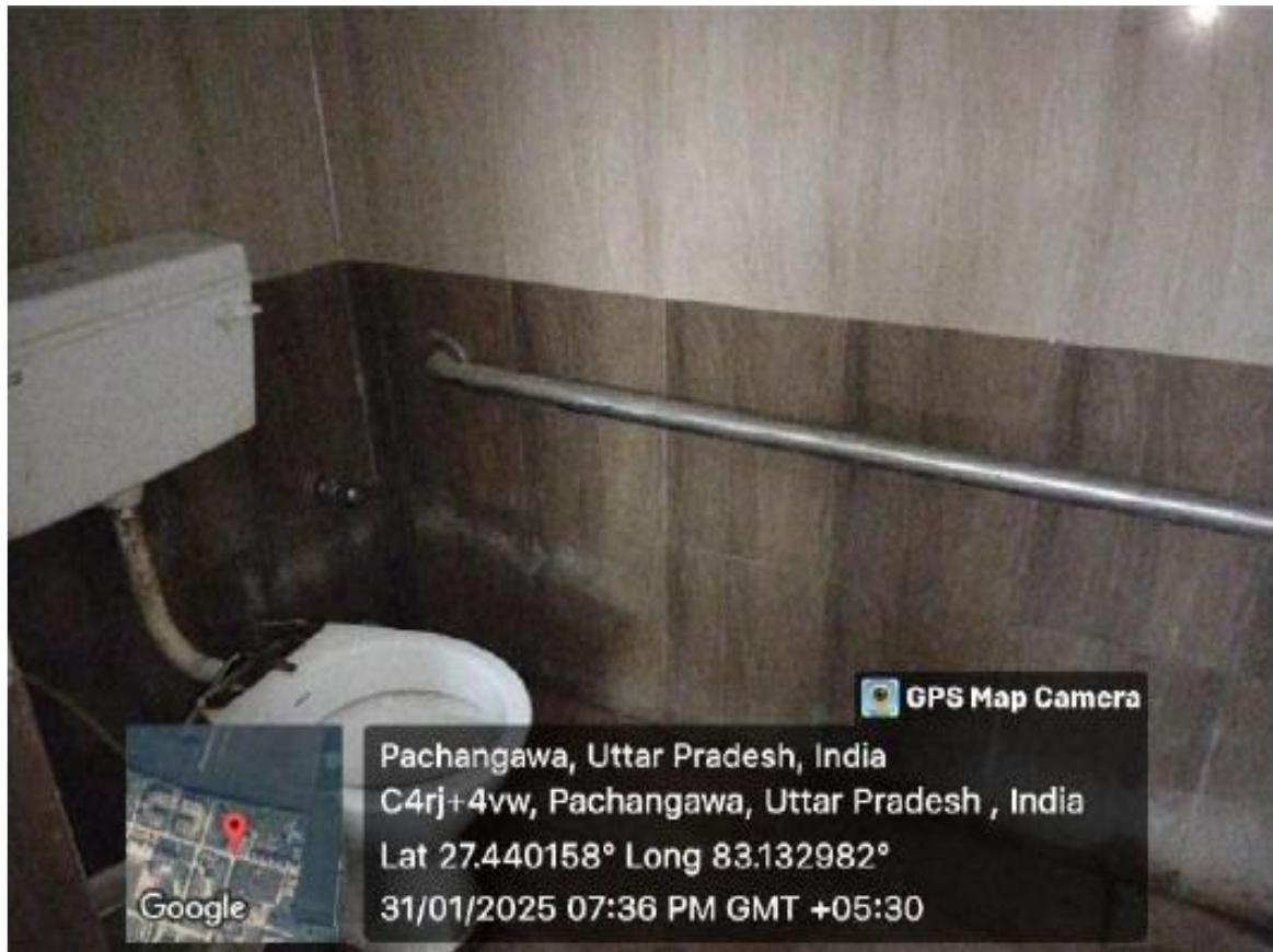
Figure 3.5.4: Grab bars in washrooms
