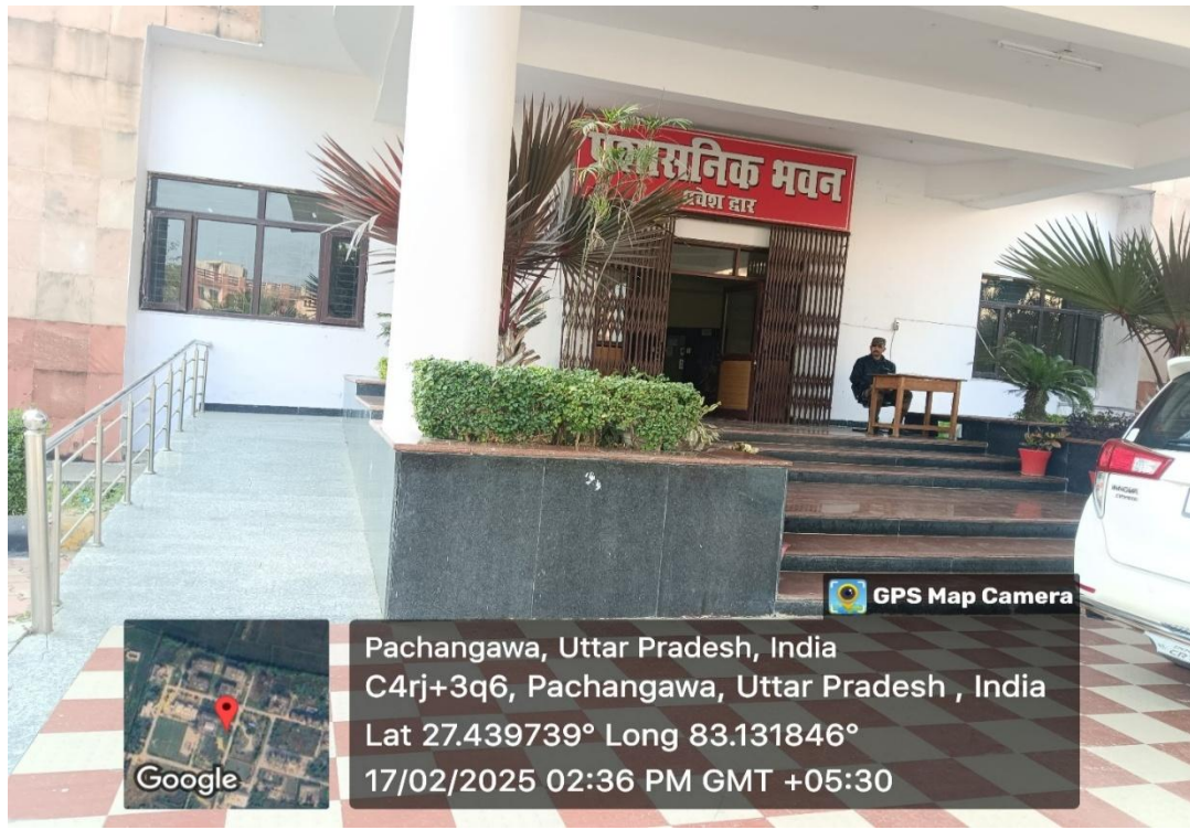
Figure 3.5.2: Ramp in the administrative building
