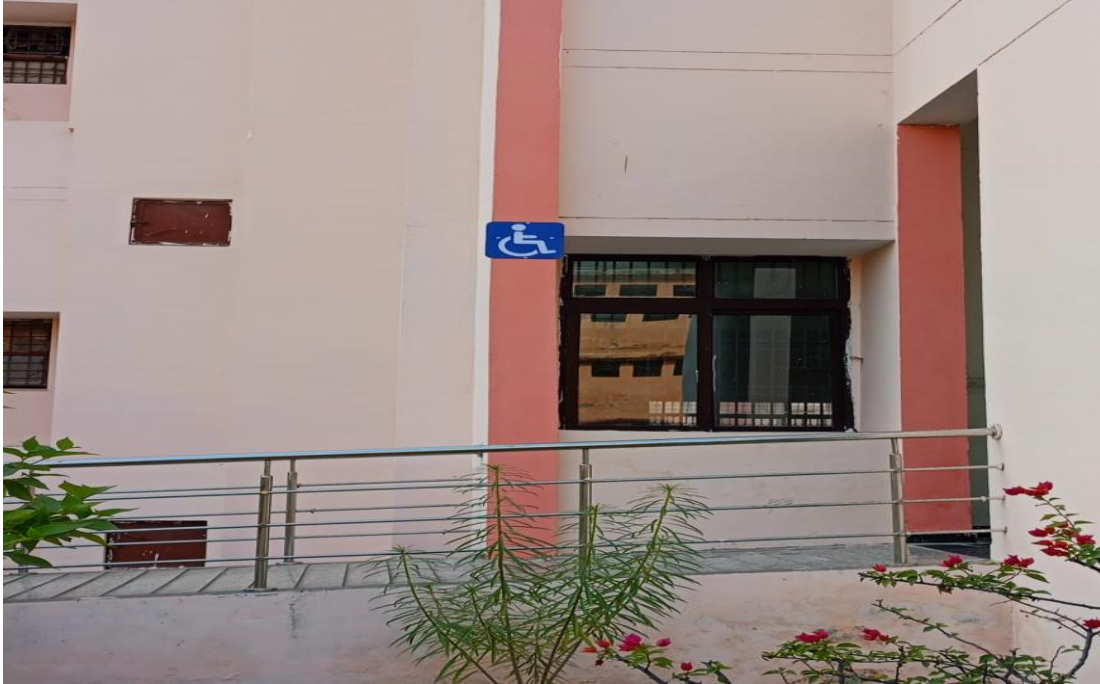
Figure 3.5.7(b): Ramp Signage
